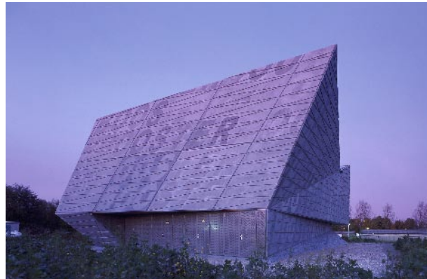
Booster Pump Station East, Amsterdam (2005)
