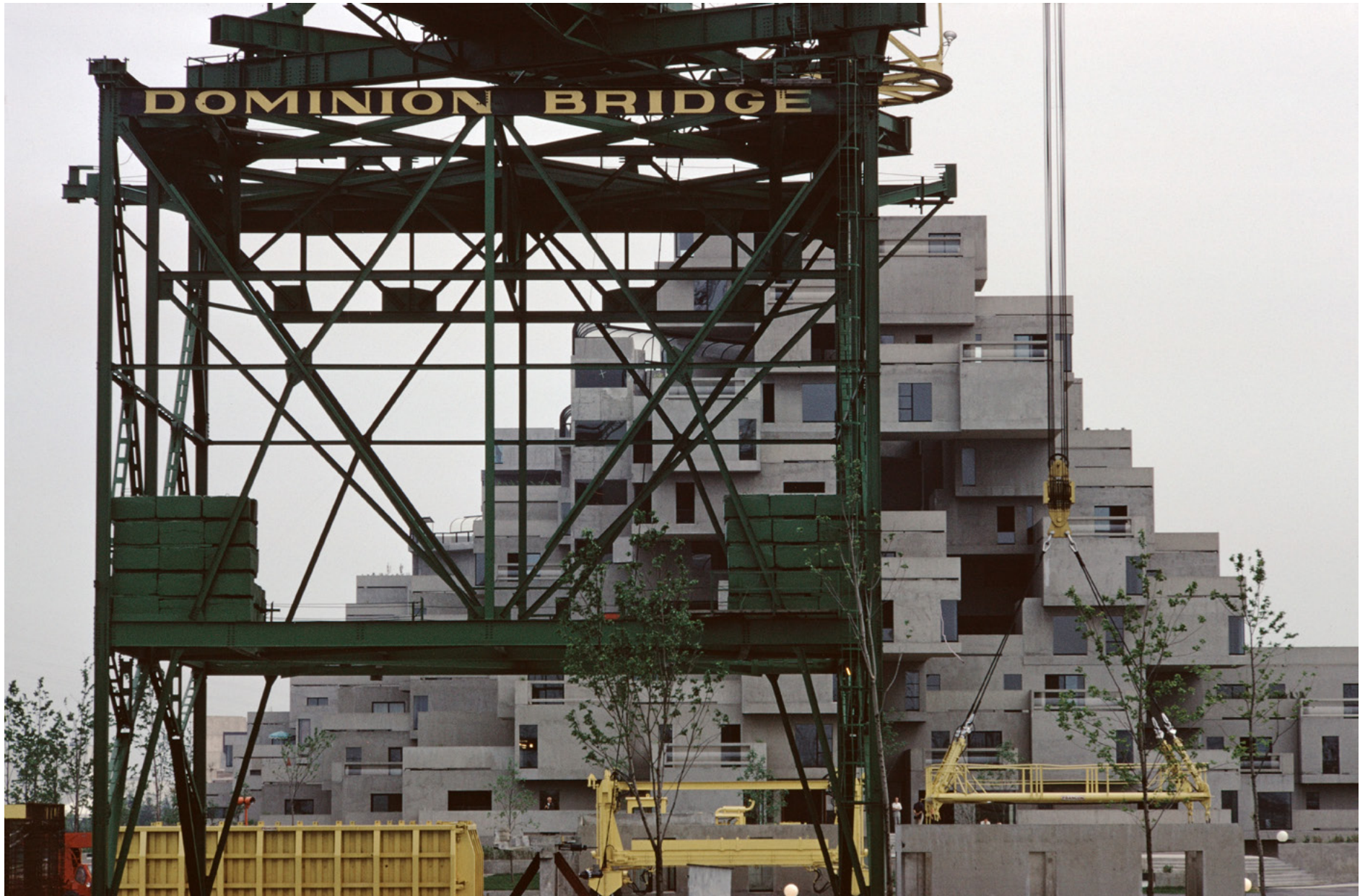
Moshe Safdie, Habitat 67 under construction, Cité du Havre, Montréal, Québec, 1967, aus: Observation Is a Constant That Underlies All Approaches , Lars Müller Publishers, 2023, S. 208, © Phyllis Lambert
