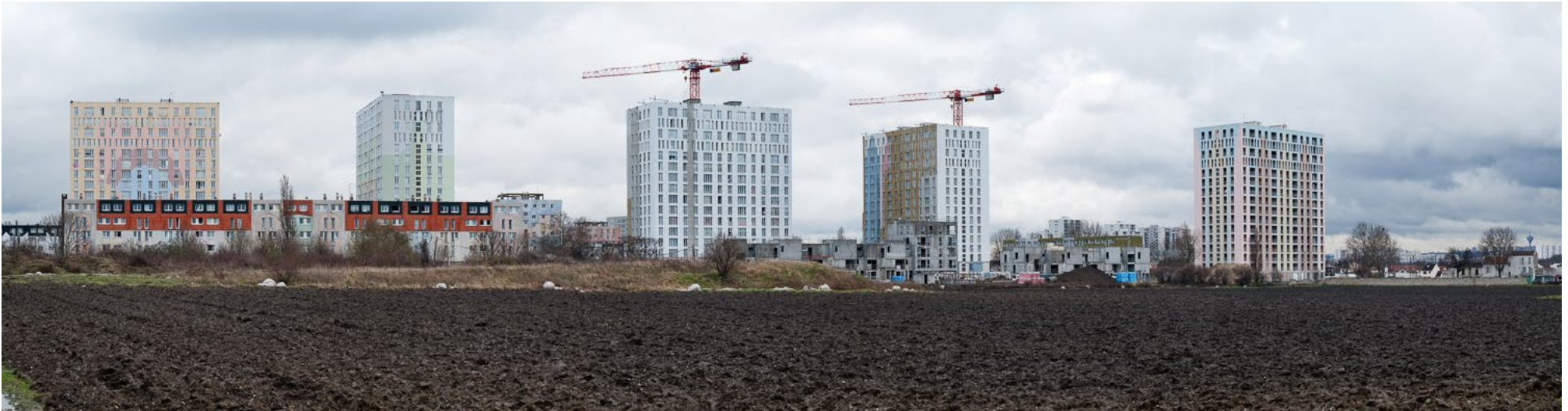
Das Grand Ensemble Le Clos Saint-Lazare in Stains, Seine-Saint-Denis, Foto: Martin Argyroglo
